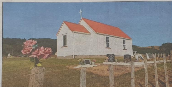
Samuel Marsden Māori Anglican Church, ready for another century after renovations.
