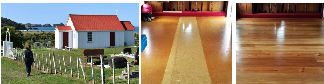
Illustration 3: Samuel Marsden Memorial Church at Matauri Bay. Floor replacement from chipboard (before) to farm-tōtara (after) from a farm site nearby
